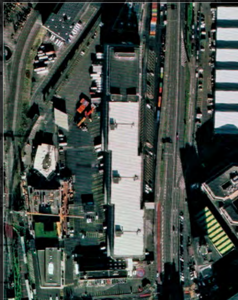
Satellite view of Geneva Free Ports and Warehouses, in Geneva, Switzerland. The freeport's management guarantees discretion, but visitors have described stockpiles of gold, cigars, fine wines and art inside the high-security compound.
